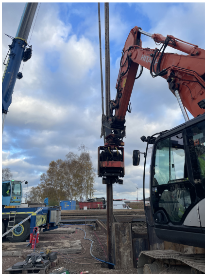
(a) Spontinstallation, del 1.
