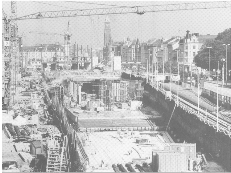
Figur 5.6 – Cut-and-coverprincip. Knutpunkten
